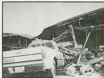
Blast collapsed cinder-block structure three blocks to the northwest of federal building. Some 75 buildings in area were rendered uninhabitable by explosion.
